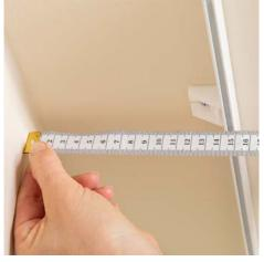
**5.** Decide how far from the wall you want the rail to be installed. Screw the rail directly into the ceiling.
